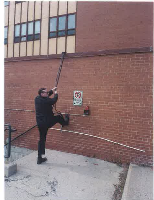
Wire allowing for easy access to the roof
